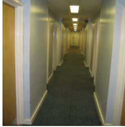
Pre-existing condition Errol St building
