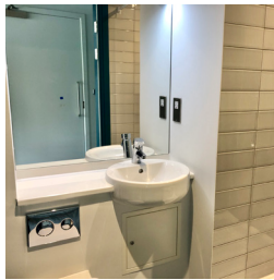
Landaid House new kitchens and bathrooms
